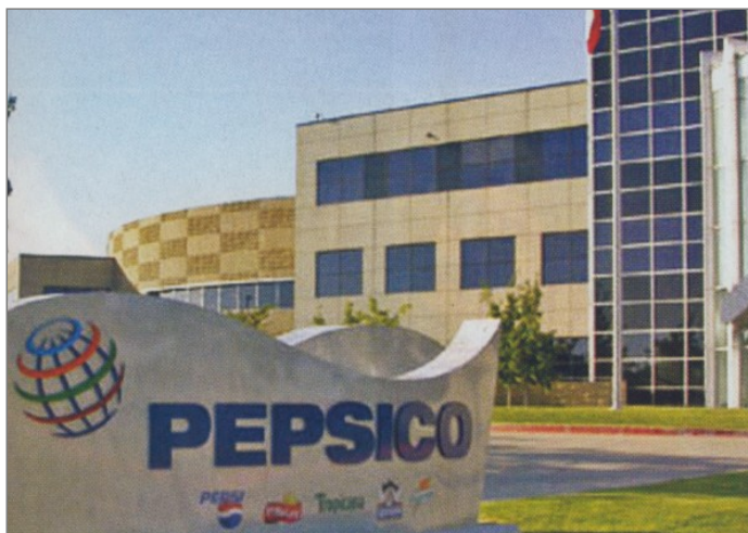
(Above): This 27-acre site at Plano, an affluent northern suburb of Dallas, Texas is the home of PepsiCo's Information Technology Division and the Frito-Lay international management team. This modern 284,000 square feet building houses 1,100 employees
